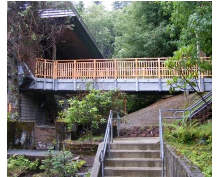
Ketchikan Campus, Connecting Bridge between Ziegler and Paul Building Photograph by UAS
