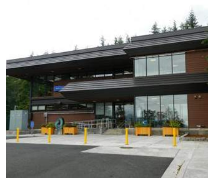
Ketchikan Campus, Ziegler Building Photograph by UAS
